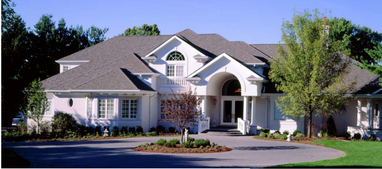
The front elevation of the Millennium II house.
