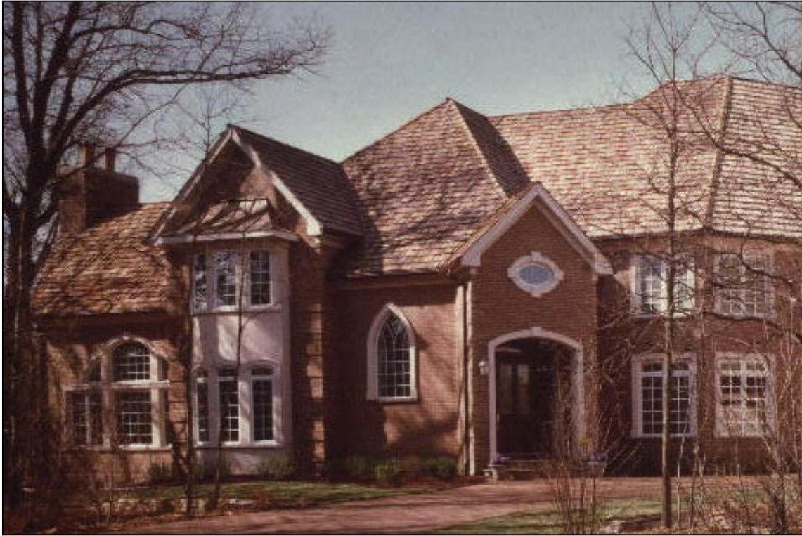
Sevon used EIFS to add detail to window details in the largely brick exterior. The custom mahogany door in the entry measure 2 1/2" thick.
