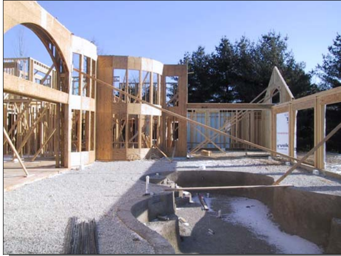
The indoor pool under construction at the Millennium II House
