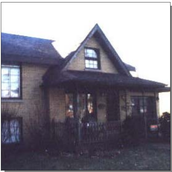
Front elevation—before renovation.
