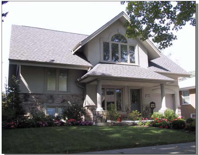
Front elevation—after renovation.
