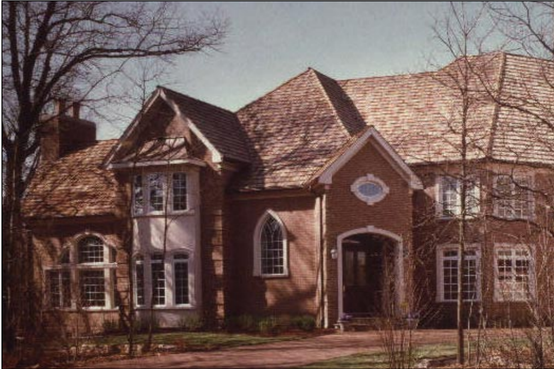
Sevon used EIFS to add detail to window details in the largely brick exterior. The custom mahogany door in the entry measure 2' _" thick.
