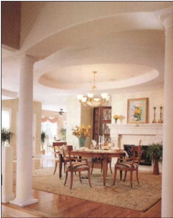
A “racetrack” soffited ceiling in the dining room defines the space. Columns and rounded drywall corners make spaces flow.
